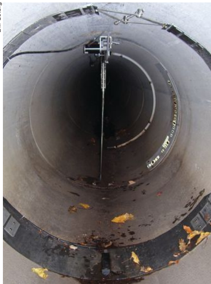
Inside a storm sewer
